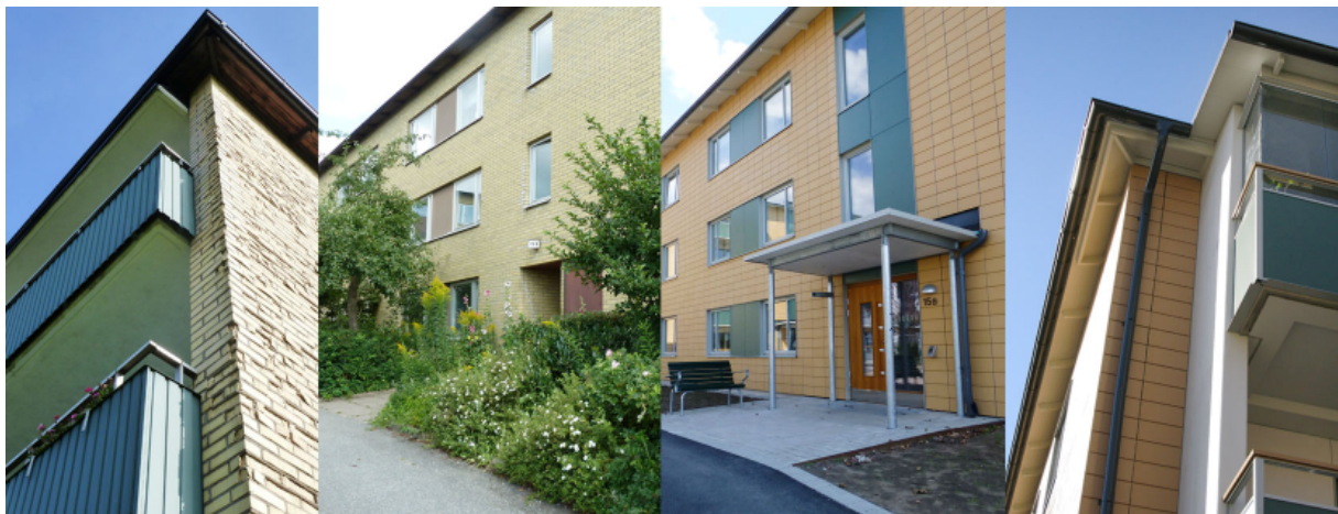
Figure 1: Brogården façades, balconies and entrances before and after retrofit. Photo: AB Alingsåshem
