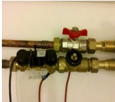
Figure 2: Heat sensor
